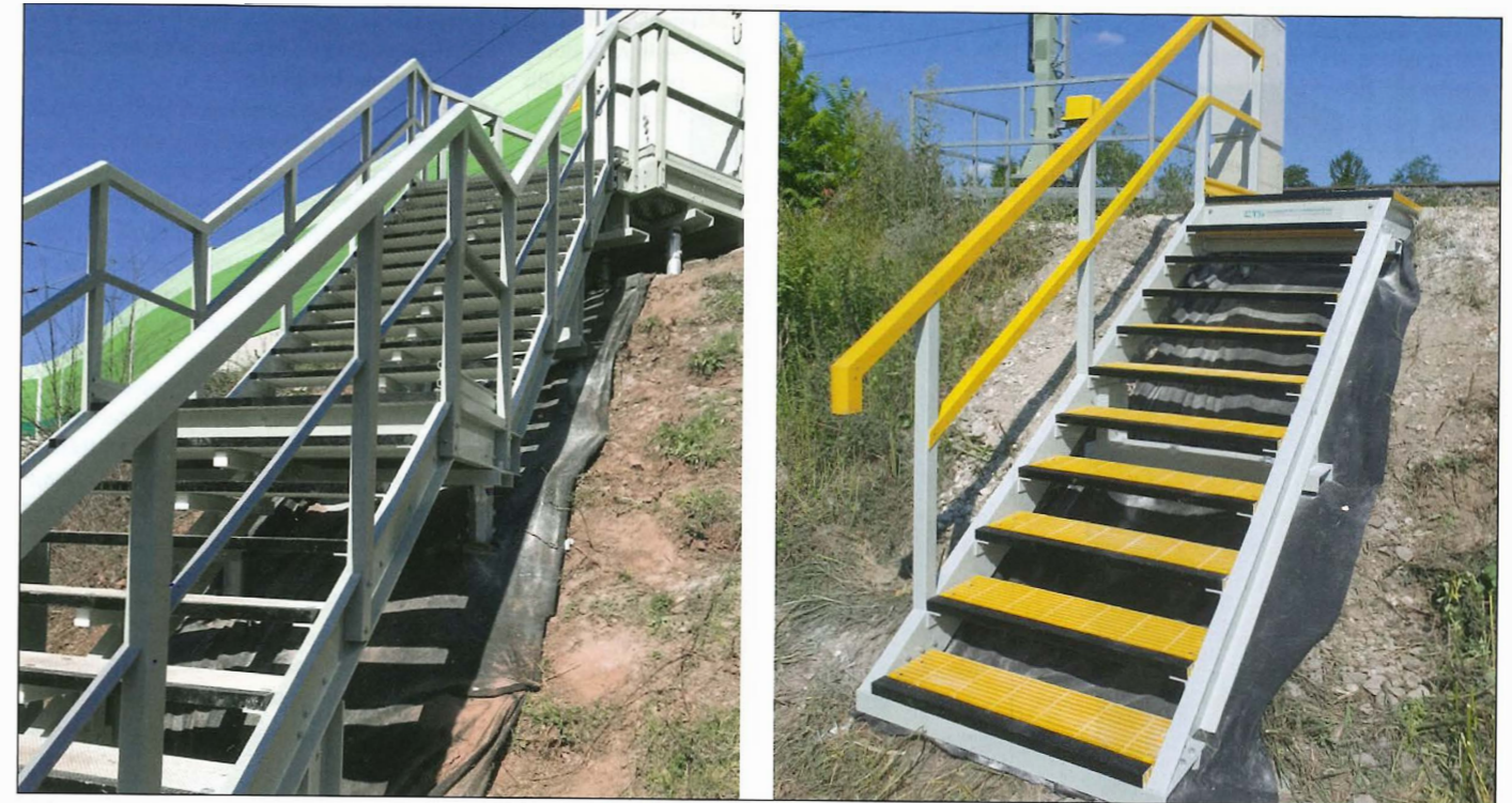
Graphic 2: embankment stairs resting on ground screws
