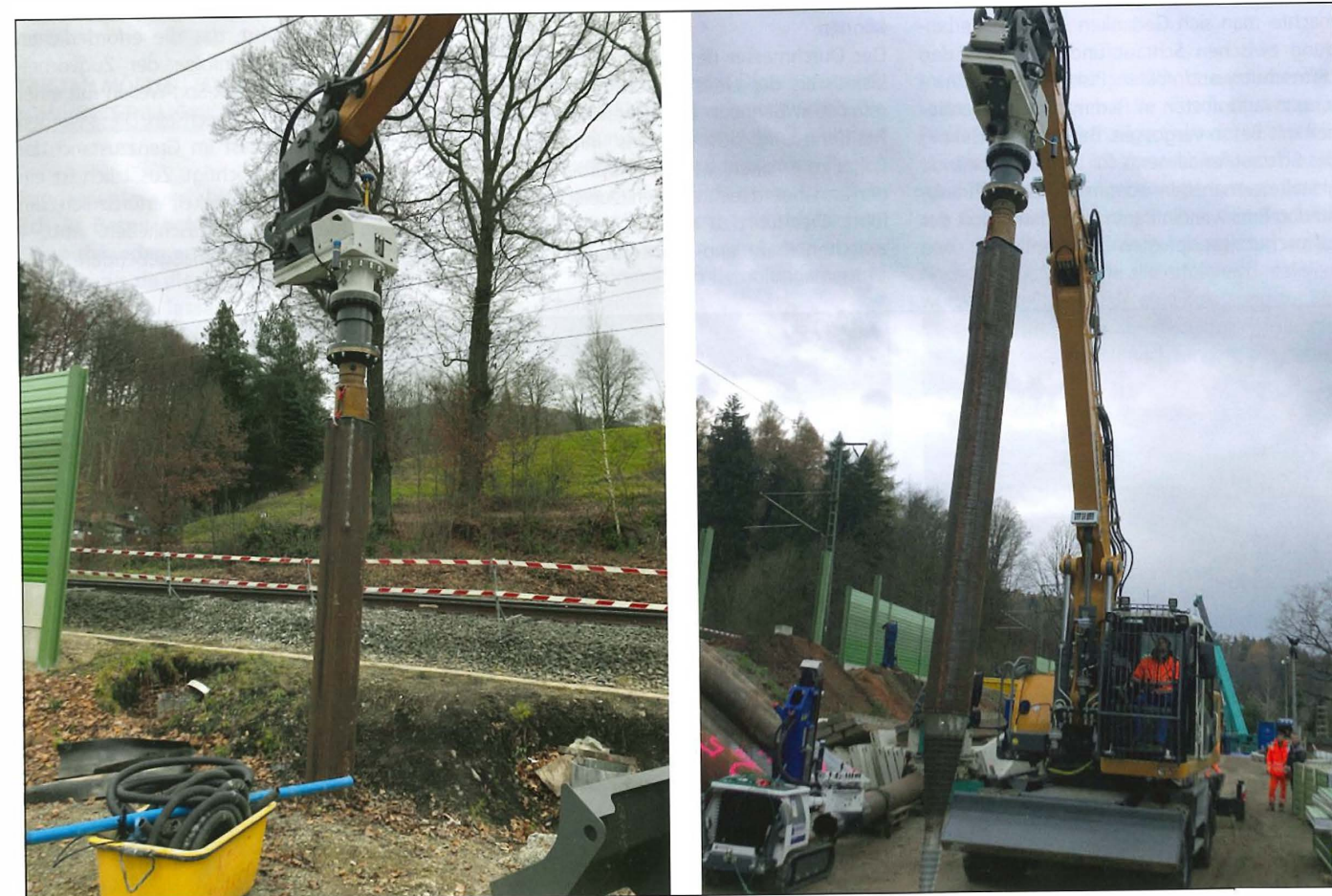
Graphic 5: test installation of ground screws
