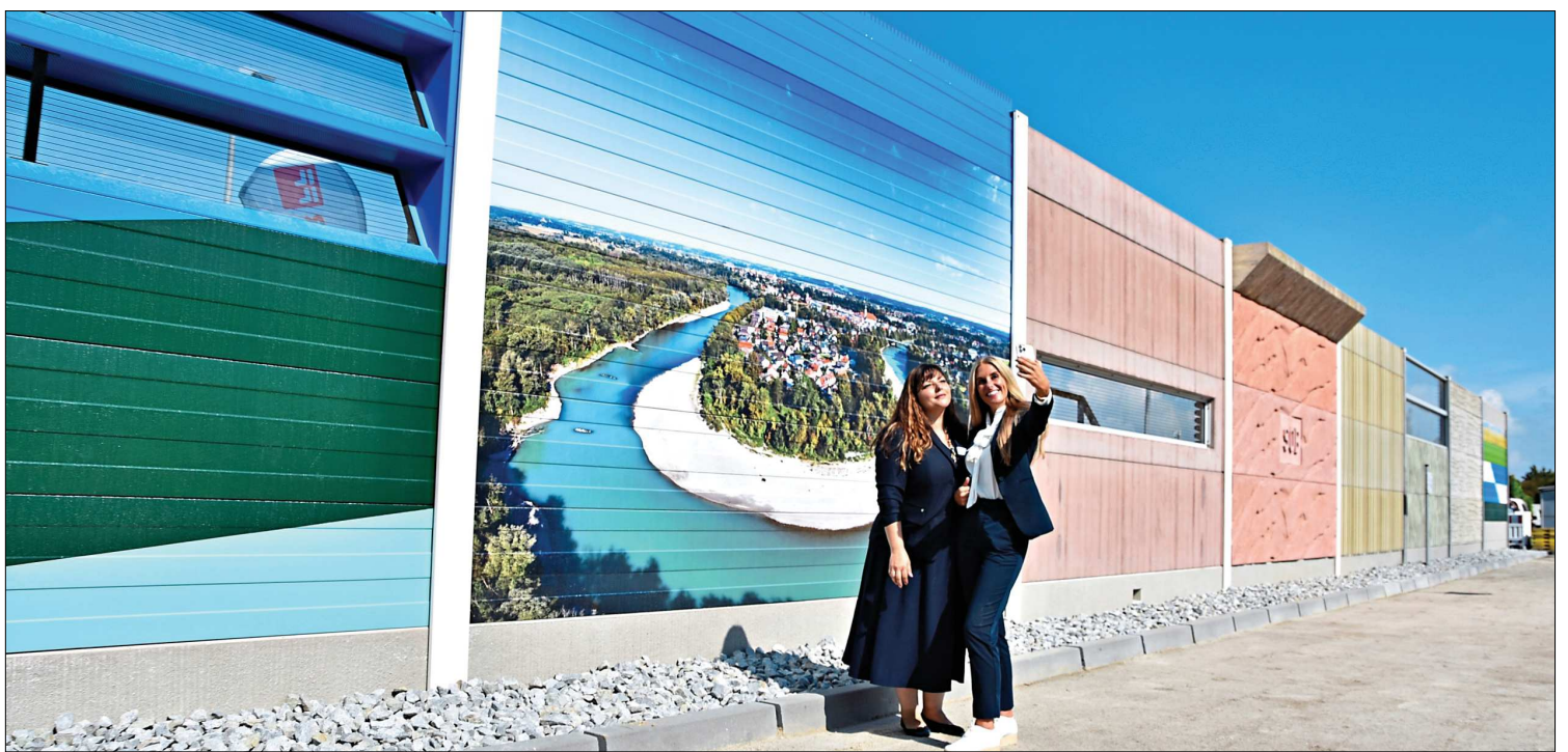
Already one of the most popular places for selfies: the "exemplary noisebarrier" with a top-down view of Mühlendorf
